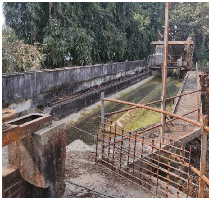
Figure 3 Grit Chamber to be used after replacing the Travelling Bridge.
