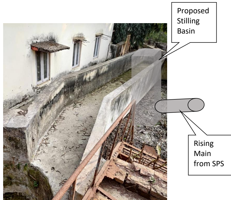
Figure 4 Proposed Stilling Chamber at the end of existing straight channel.
