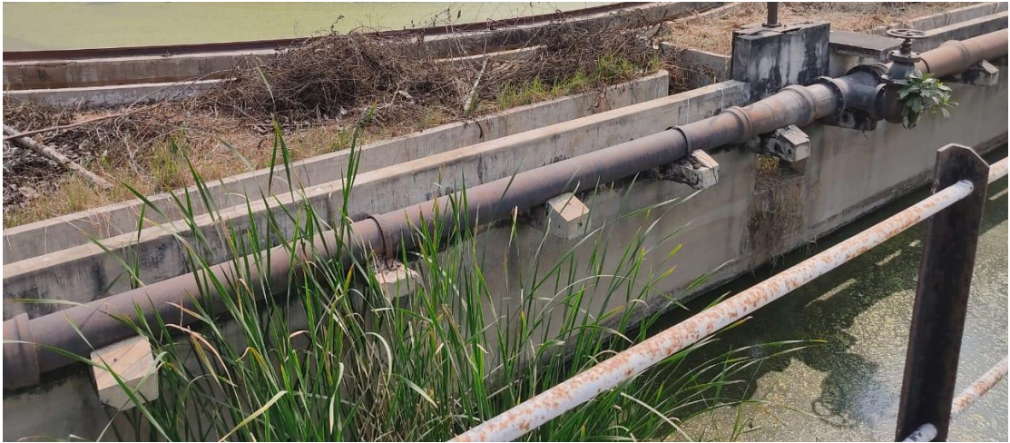
Figure 11 Existing Return Sludge Line
