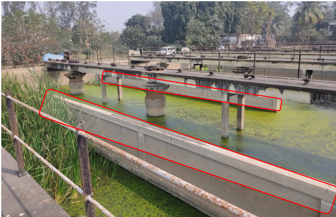
Figure 9 Existing Aeration Tank showing baffle walls in red marks.
