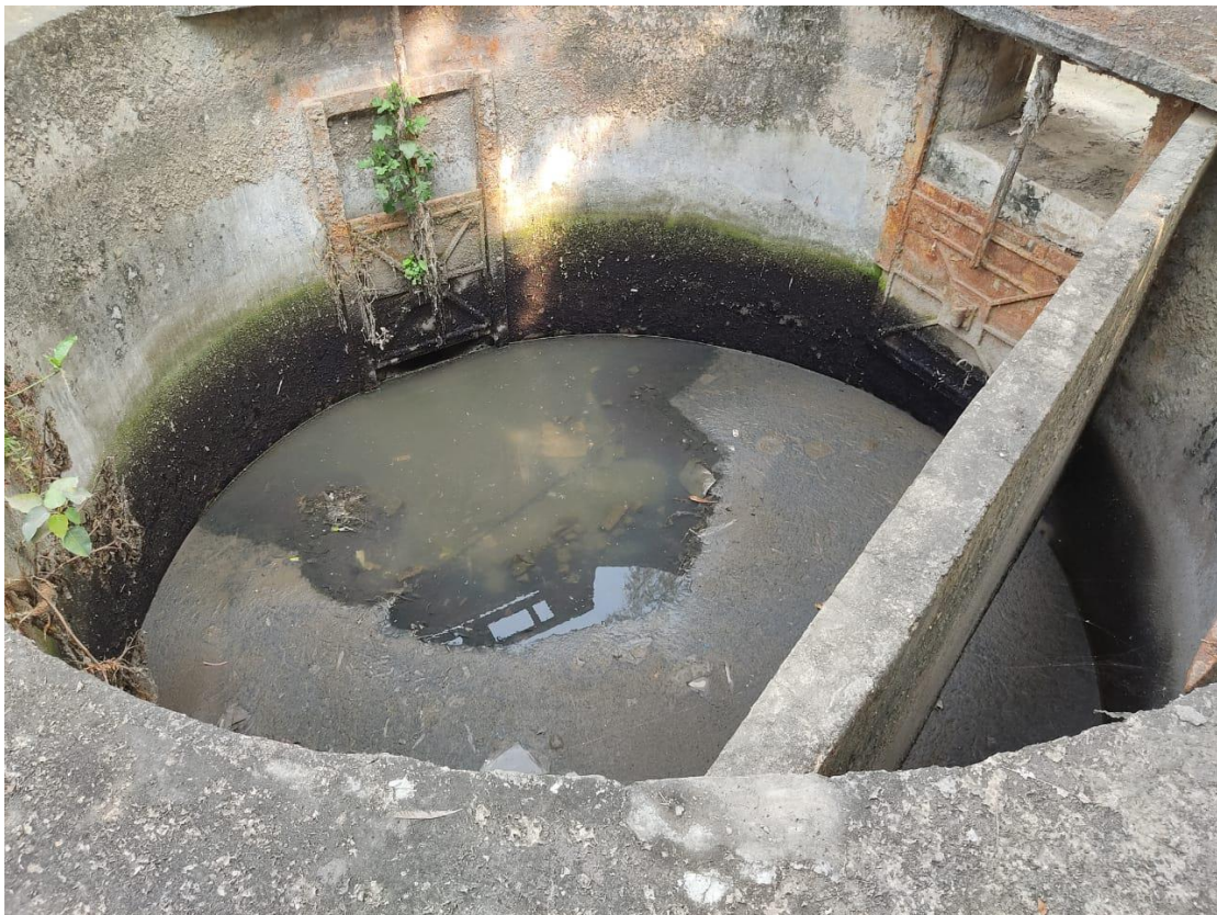
Figure 1 Existing Stilling Chamber which shall be demolished
