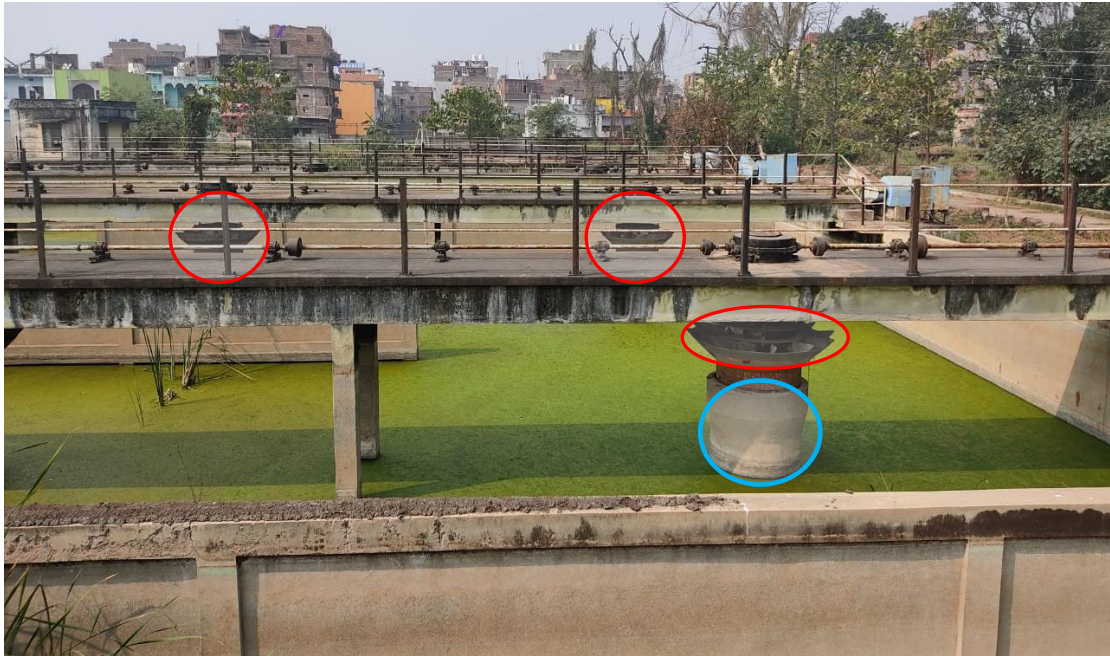
Figure 8 Existing Aeration Tank showing surface aerators (red circles), pedestals in blue circles. Pedestals shall be demolished.
