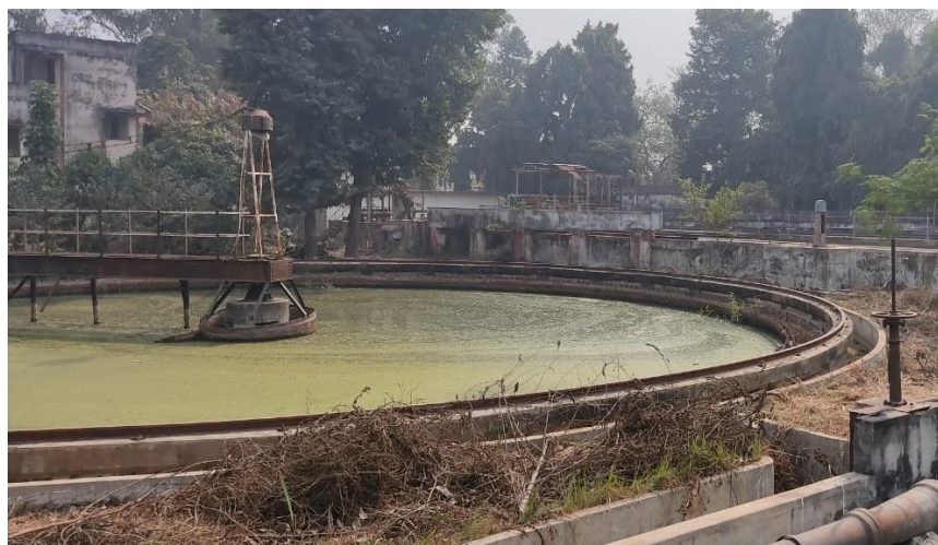
Figure 7 Existing Primary Settling Tank (PST) to be used as standby SST.
