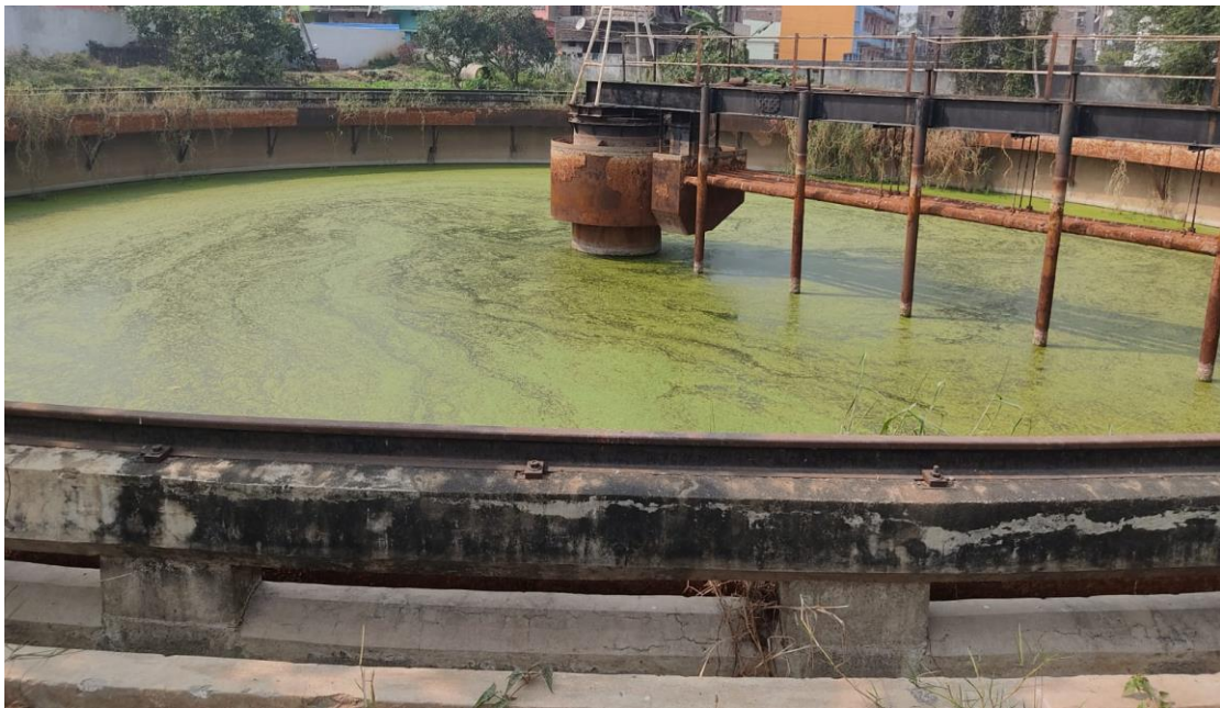
Figure 10 Existing Secondary Settling Tank shall be used after replacing all the electro-mechanical items.
