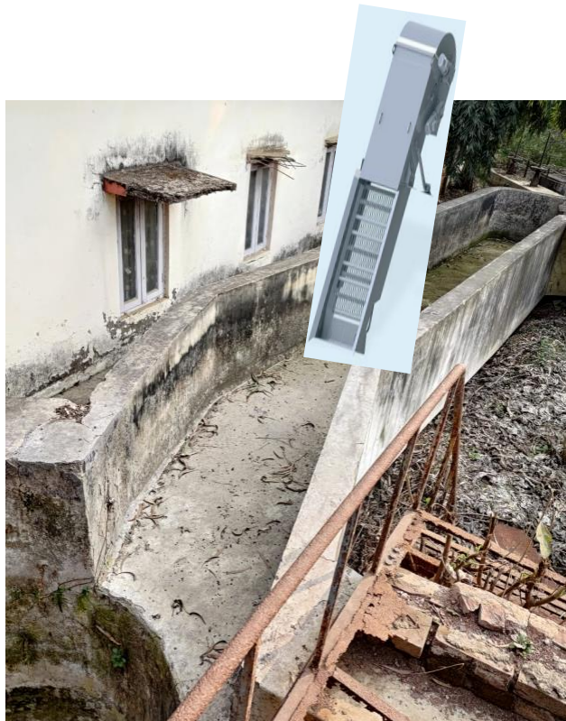
Figure 5 Proposed mechanical rake type screen after Stilling Chamber to be installed in the straight channel.
