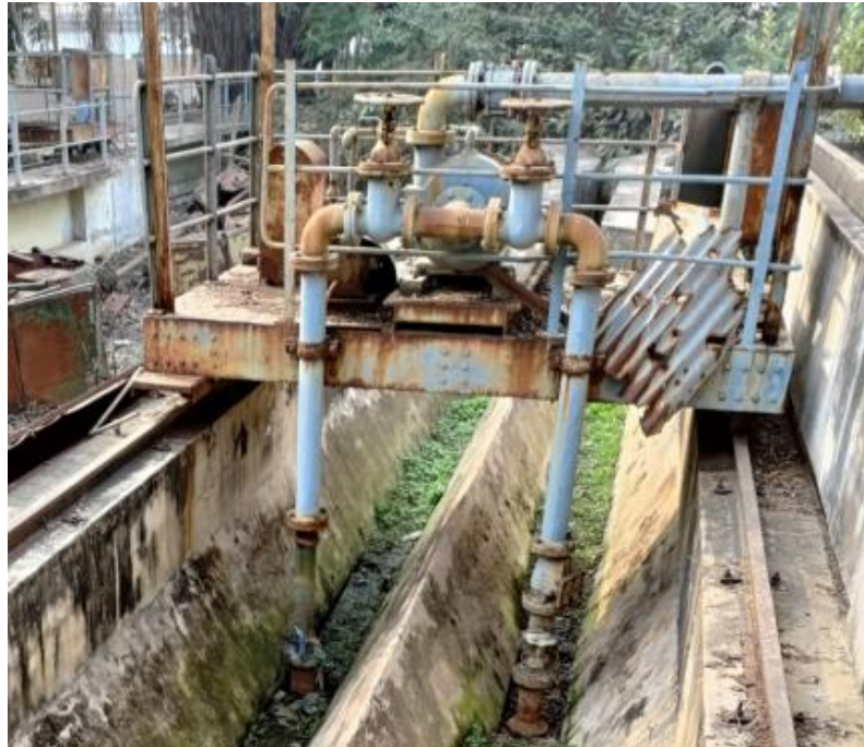
Figure 2 Travelling Bridge type grit removal mechanism which is to be replaced with new one.
